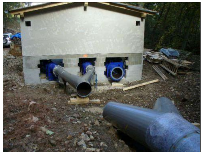
Reconstruction of Small Hydropower Plant
